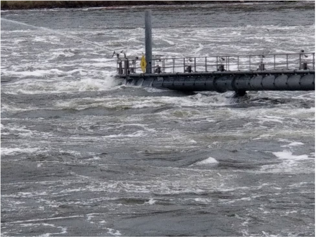
Figure 1: Lower Granite outfall pipe on June 13, 2022.
