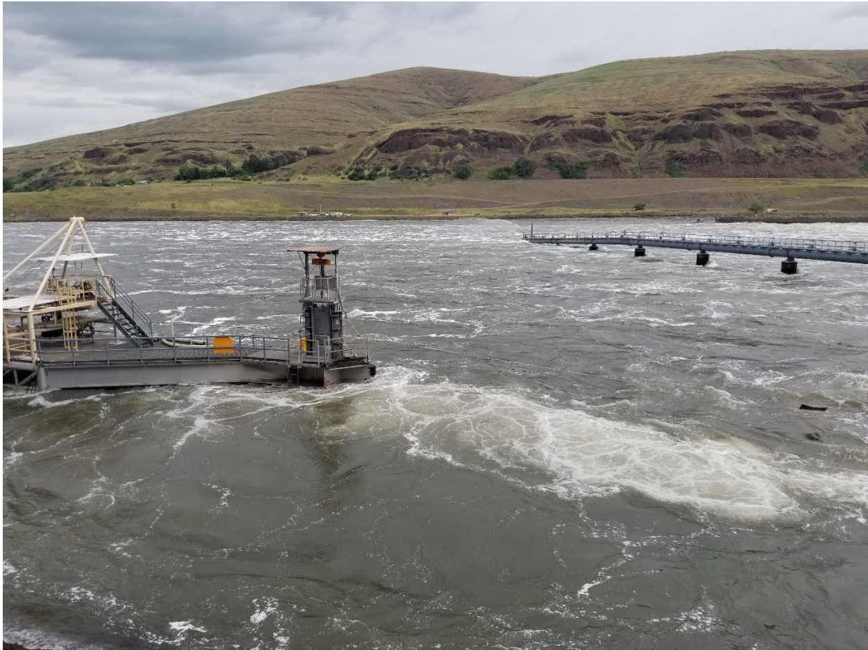
Figure 2: Lower Granite Barge Loading Dock on June 13, 2022.
